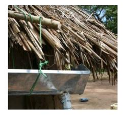
Wooden supports can be used and are more solidly positioned. Either they are treated with termite protection or they are replaced when necessary.
