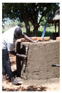
The DRIP tank is a fired brick built cylindrical tank standing on a base of approximately 1.5m diameter.
